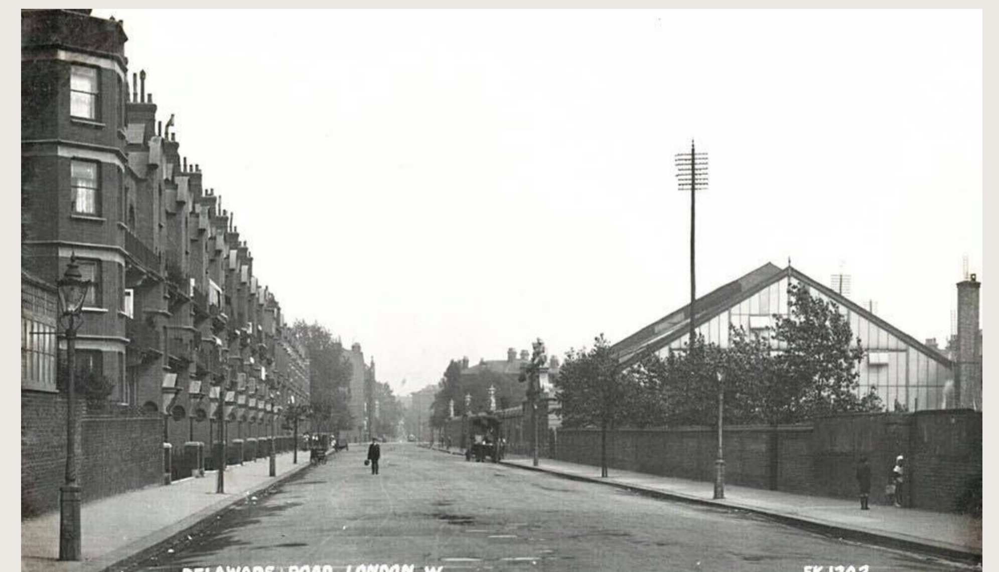
DELAWARE ROAD, LONDON, W. FK 1202 DELAWARE ROAD, 1910
